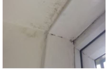
Example of mould / damage due to cold air behind plaster board or window reveal
