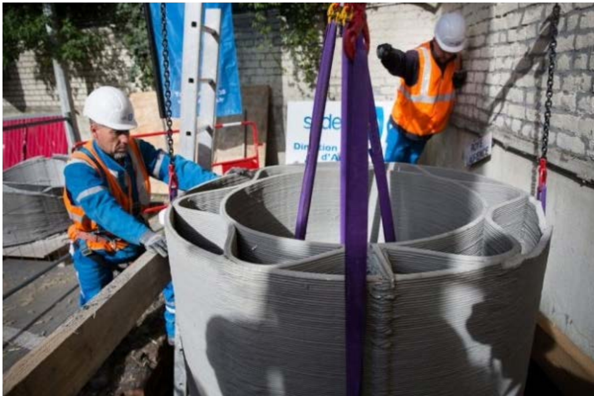
Figure 4: 3DP Inspection chambers in Roubaix (Source: XtreeE )
