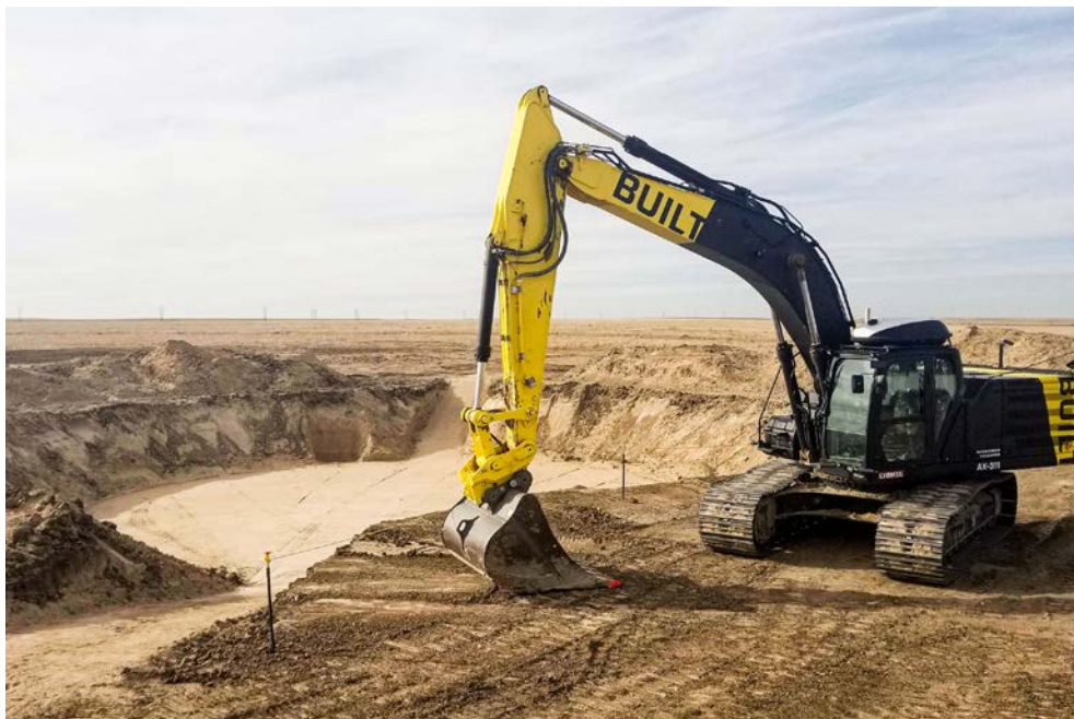
Figure 6: A completed wind tower foundation using a robotic excavator (Source: Built Robotics )
